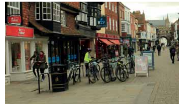
Uncoordinated street furniture and signage undermine the quality of the High Street.
